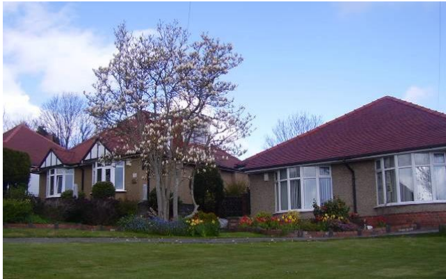
Bungalows offer accessible accommodation. Any roof alterations must be carefully considered
