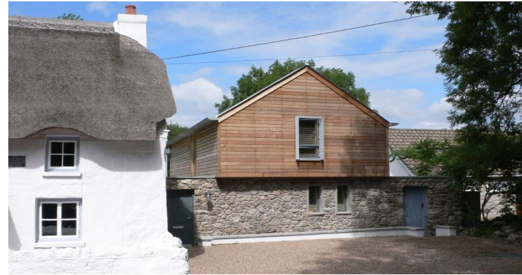
Contemporary extension to a thatched cottage, Oxwich (Winner of several 2006 Design Awards)
