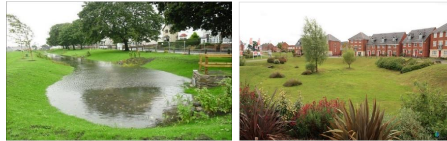
Filled detention basin served from swale and separate underground SuDS outlet pipe (left) and a dry detention basin with planting (right) adding to local character, biodiversity and providing amenity space
