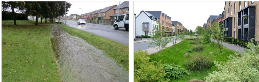
Simple grassed swales convey water during wet weather (left) and a vegetated street swales (right) can improve biodiversity and street character
