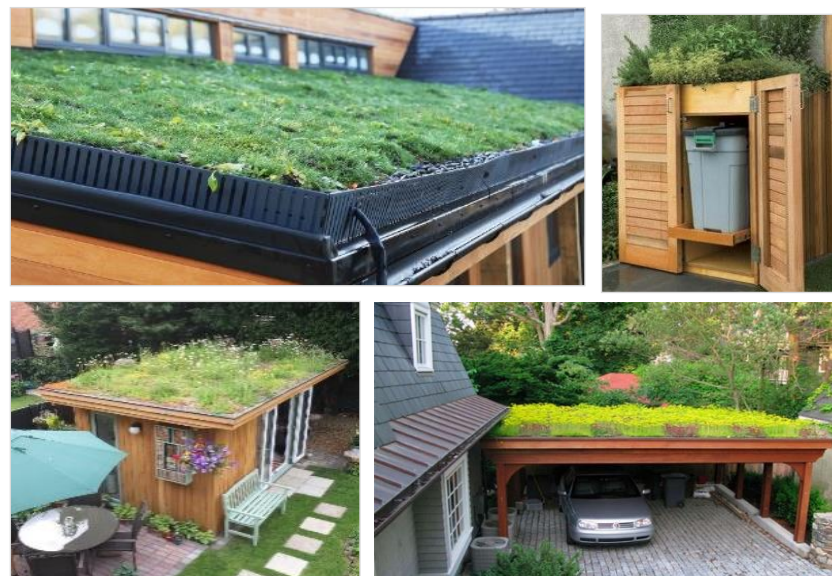
Green roofs can be applied to a number of flat or shallow pitched structures - extensions, sheds, stores and garages or car ports
