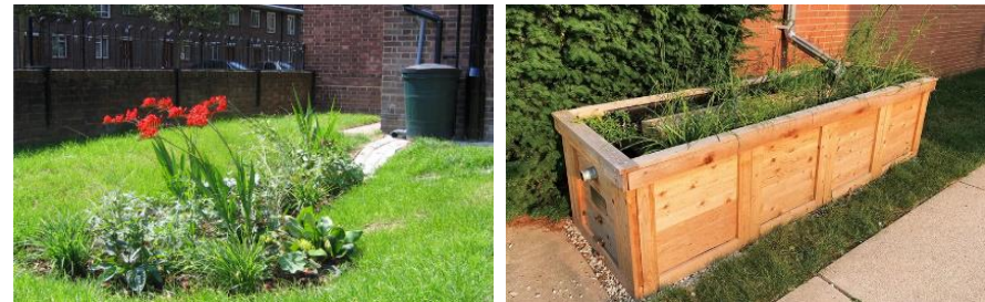
Rain gardens can be surface level and include water butts (top) or provided as planter boxes (bottom)
