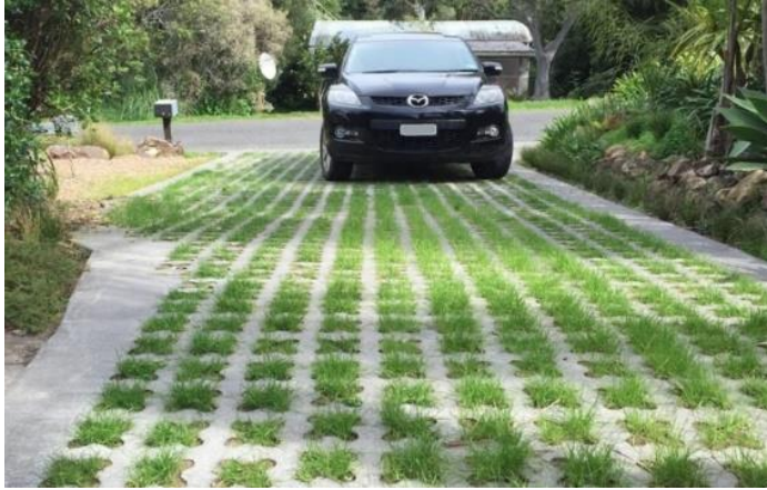
Permeable block paving driveway with grass
