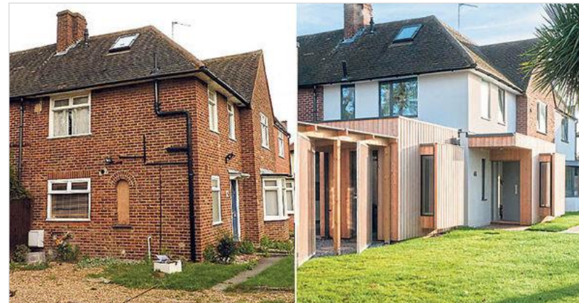
Enhancement scheme utilising contemporary extensions and render
