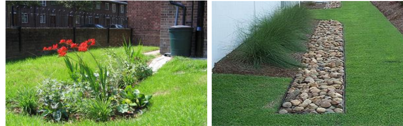
Plot level features such as a surface level rain garden (left) and infiltration trench (right) can be incorporated into developments
