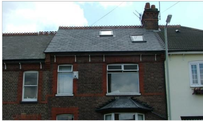
Rooflights to front roof slope
